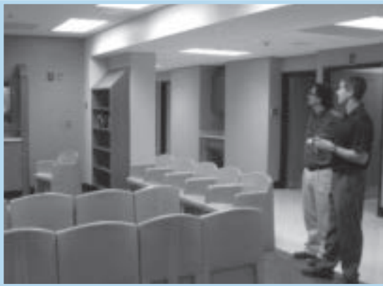
Adolescent Psychiatric Renovation - Construction
